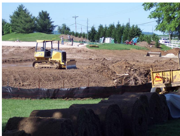
Shaping the new green and bunker.
